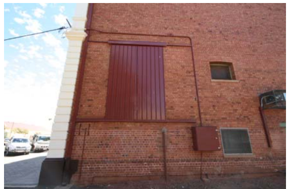
Rear Loading Doors at Boulder Town Hall
