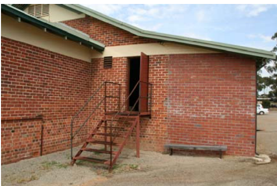
Stairs to rear of stage (Load In Access)
