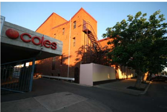
Rear 3D of Venue (Load In from Coles driveway to rear Stage)
