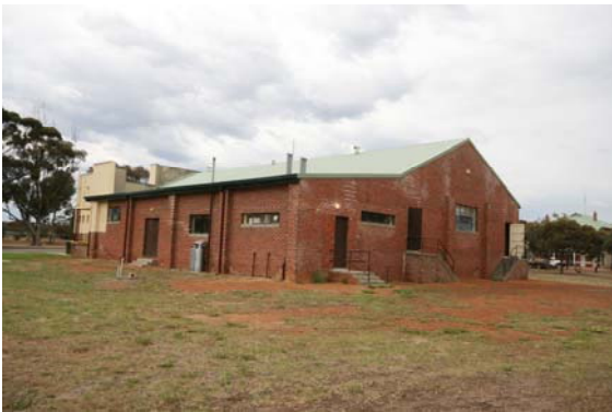
Side of Venue & Rear of Stage (Load in from Truck)
