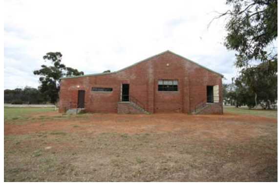
Rear of Stage (Kitchen entry through door on left)
