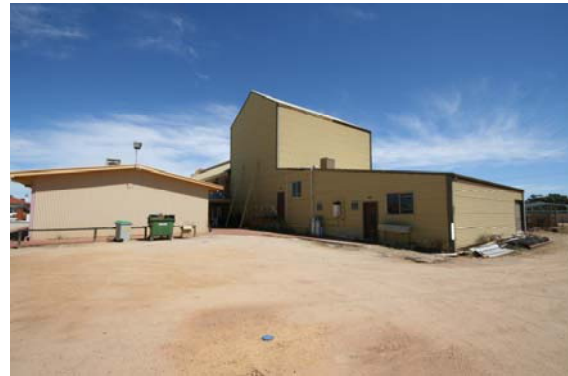
Rear of Venue (& Dressing Room doors)
