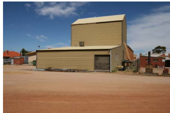
Loading Dock access at venue rear
