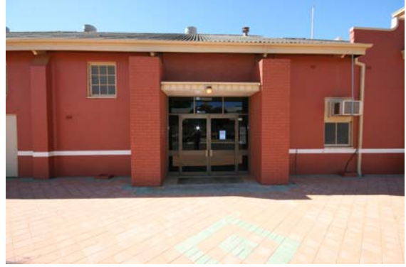
Load in access at Myers St side of venue
