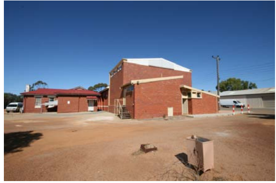
Rear of Venue (& Dressing Room doors)
