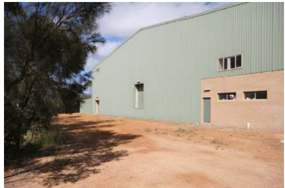
Rear of Venue & loading door (& plenty of truck/bus/company parking)
