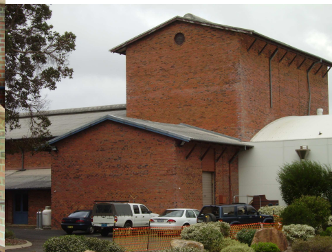
Rear truck height load-in bay
