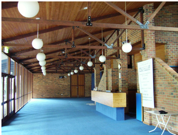
Foyer and stairs to upper balcony
