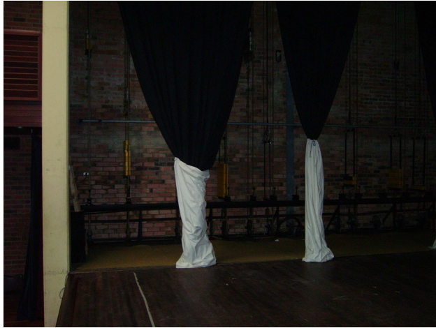
Counterweight system on stage right
