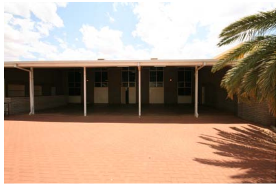
Load in access at side of venue (through double doors)
